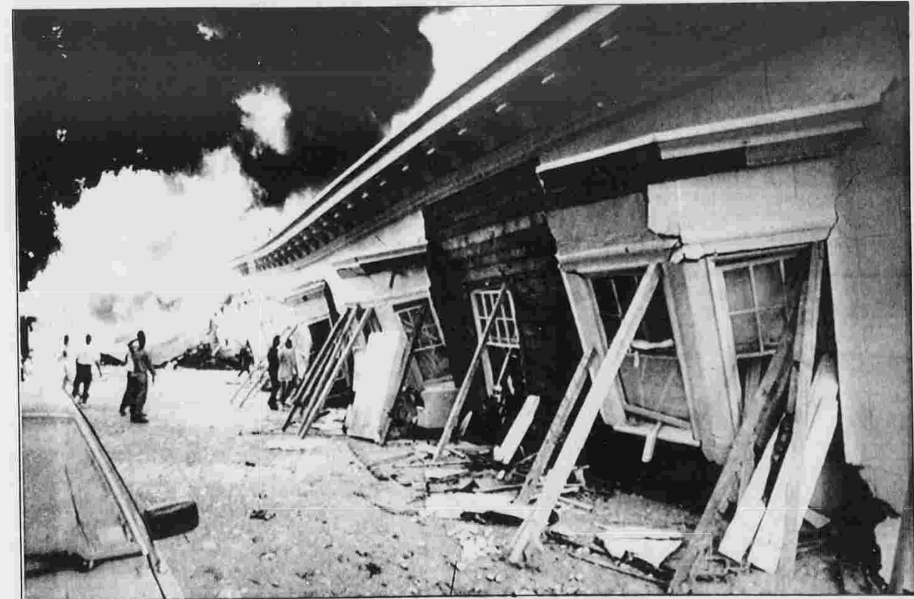
AFTERMATH — Fires fed by broken gas lines rage behind propped-up buildings.
