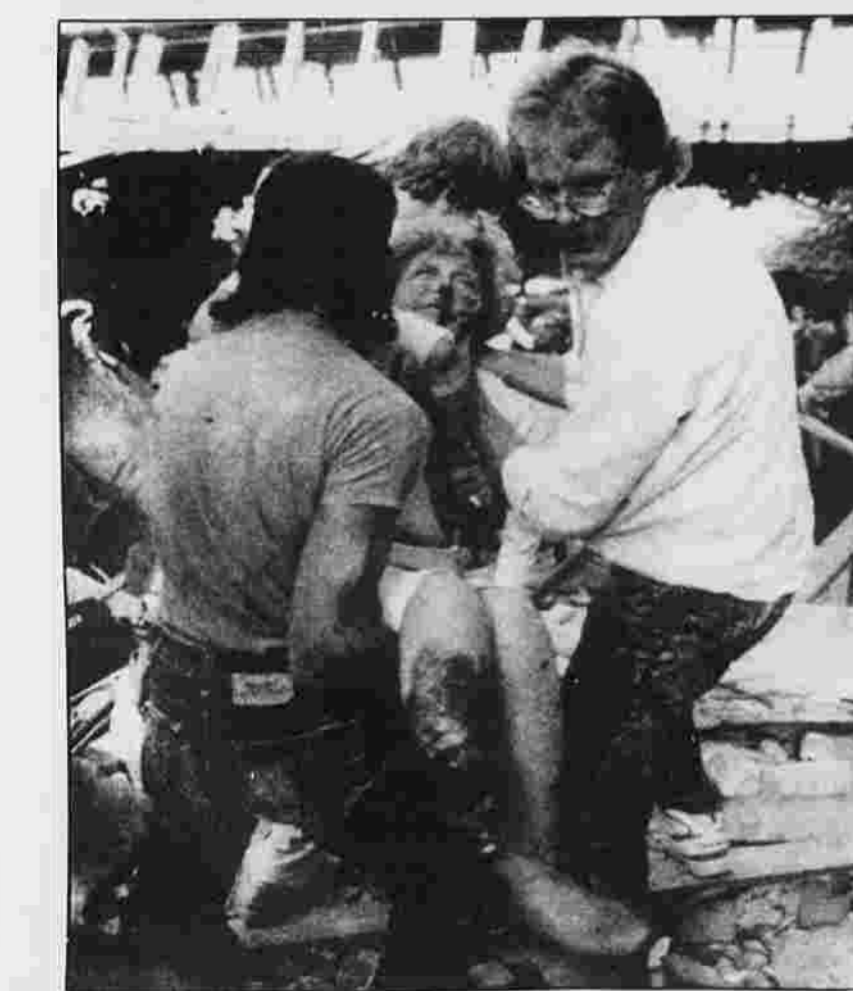
RESCUED — Survivor is carried from the rubble of a building.
